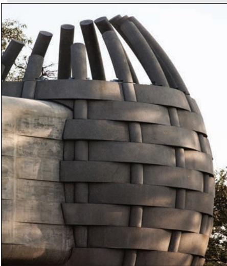
Photos Courtesy of Metro Gold Line Foothill Extension Construction Authority
